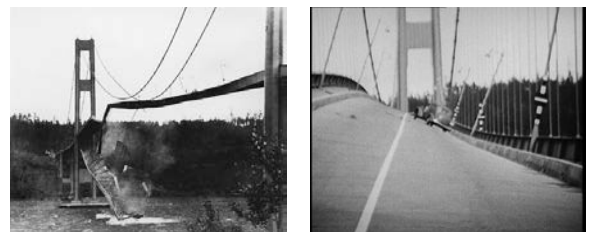
FIGURE 3. Tacoma Narrows Bridge collapsed during hard wind (The bridge opened on July 1, 1940, and collapsed on November 7, 1940).
