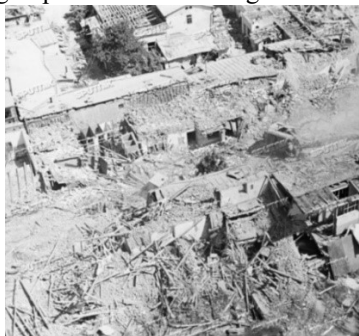
Fig.1 1966 Tashkent Earthquake Damage (by the website of https://sputnikimages.com/media/728747.html )
