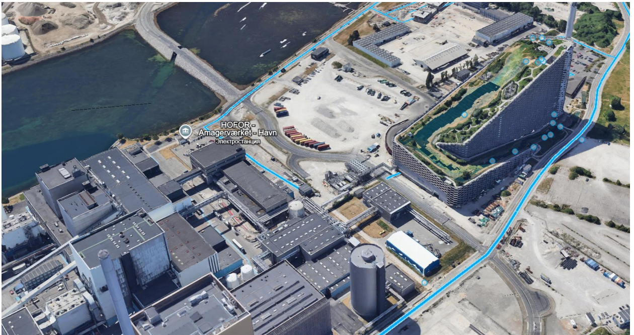
Рис.3. Amager Ressource Center (ARC)
